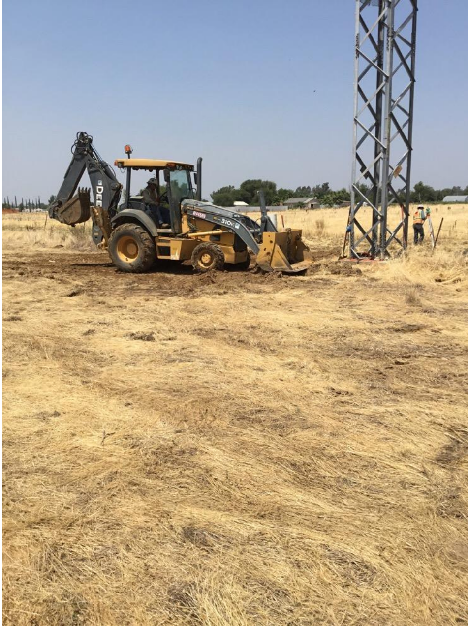
Photo 2: Backhoe preparing ground for drilling at Pole 1/17.
